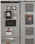
Automatic water display unit conditions as a meg-ohm meter. This automatic testing equipment replaces the hand meg-ohm-testing approach for determining whether a generator can be started safely.
