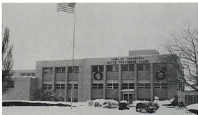
The Town of Tonawanda operates a 24 mgd potable water facility and a 30 mgd wastewater treatment plant near Niagara Falls, NY.
