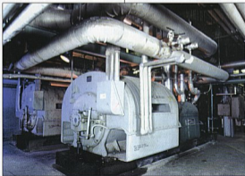
A variety of critical equipment, such as this boiler feedwater pump, is monitored to prevent motor failures and to ensure that the equipment starts without incident when a generating unit is brought into service.
