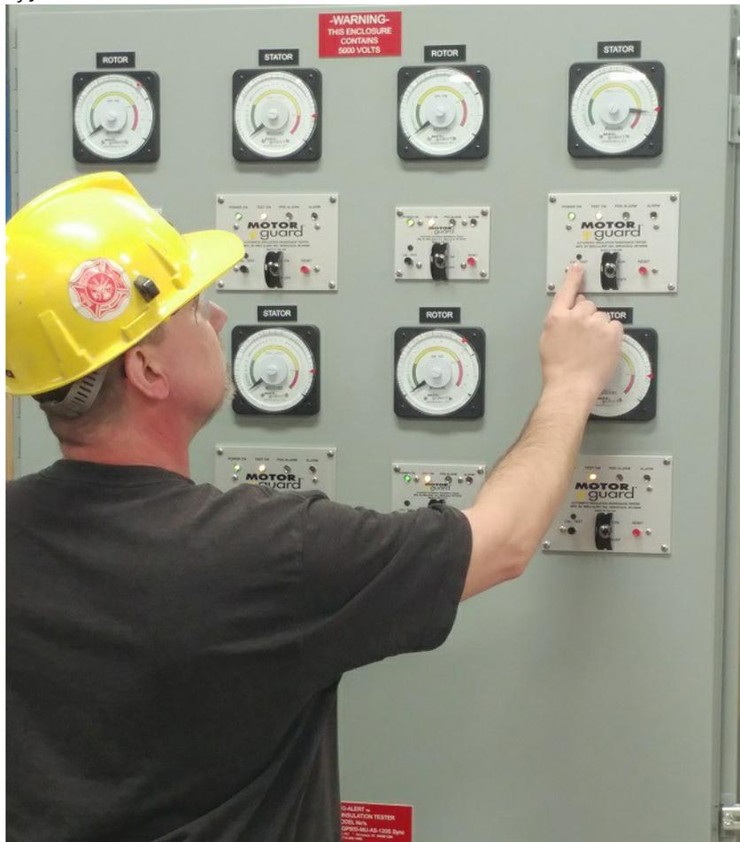
For decades, utility plant personnel have performed insulation resistance tests with handheld megohmmeters to prevent motor failures that lead to costly unplanned shutdowns, penalties and re-winding repairs.
